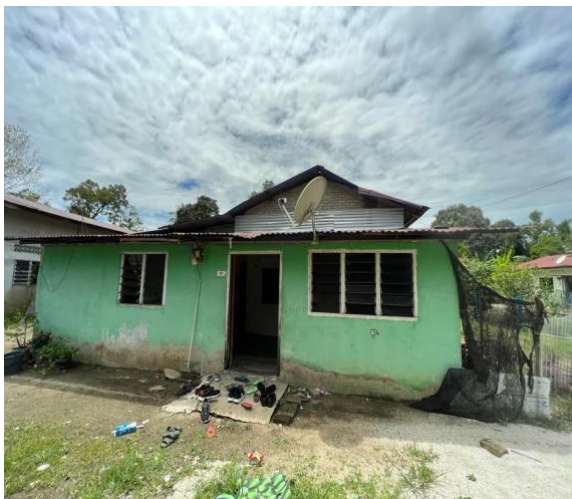
Figure 4.2: Akma's house condition
